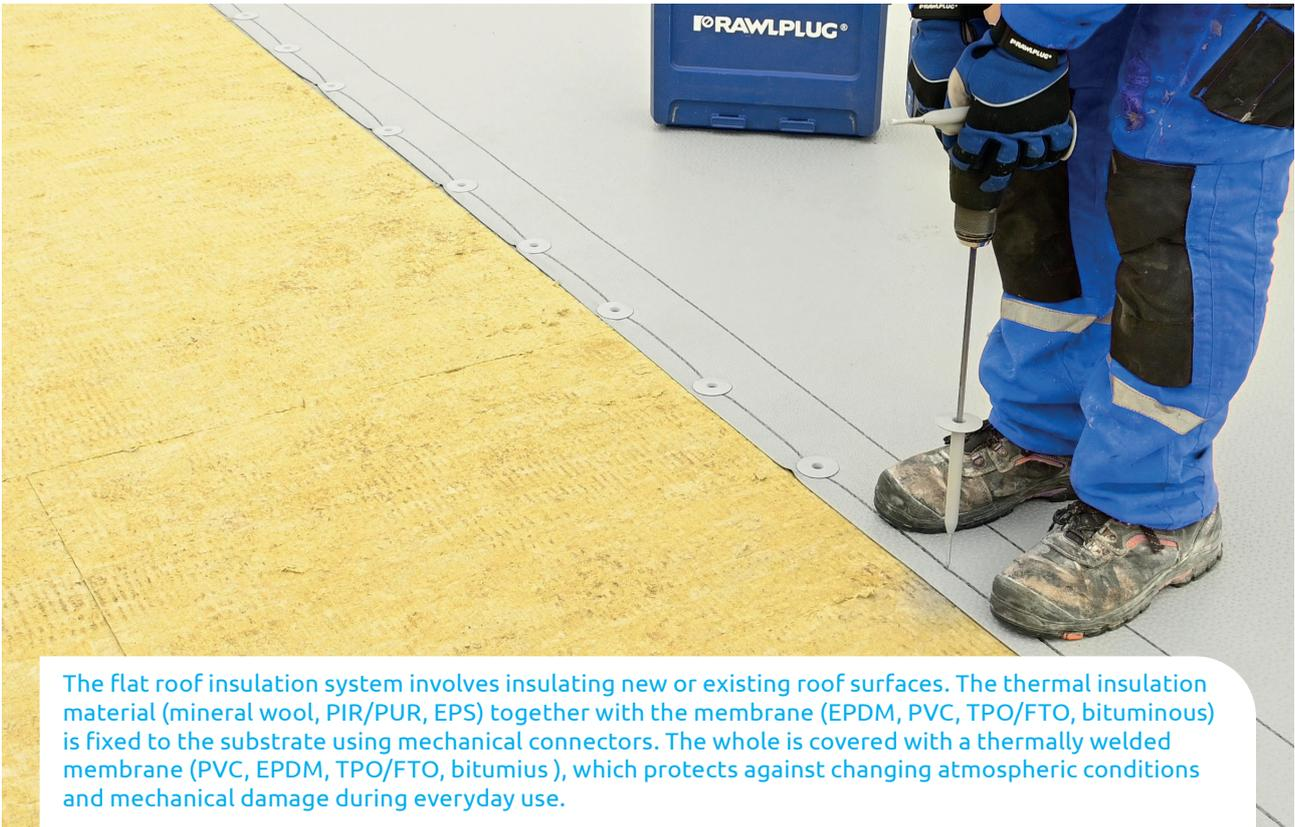
The flat roof insulation system involves insulating new or existing roof surfaces. The thermal insulation material (mineral wool, PIR/PUR, EPS) together with the membrane (EPDM, PVC, TPO/FTO, bituminous) is fixed to the substrate using mechanical connectors. The whole is covered with a thermally welded membrane (PVC, EPDM, TPO/FTO, bituminous), which protects against changing atmospheric conditions and mechanical damage during everyday use.
